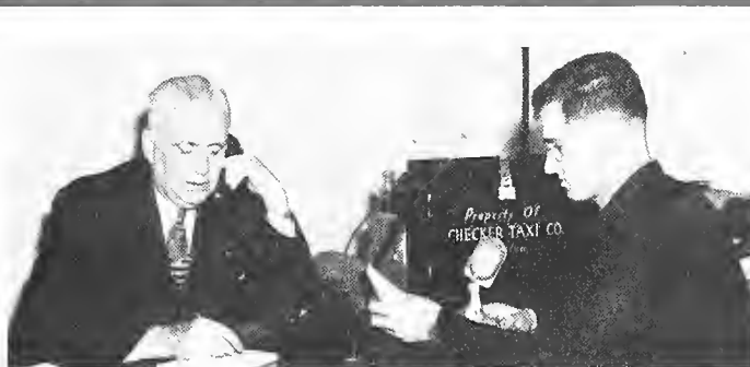
Direct radio communication with taxi-cabs in the Boston area is maintained at the Boston Civil Defense Control Center. In action are: H.L. MacOdrum (l.), Communications Officer for Taxi Cab Radio and S.M. Wolf, Dispatcher.
